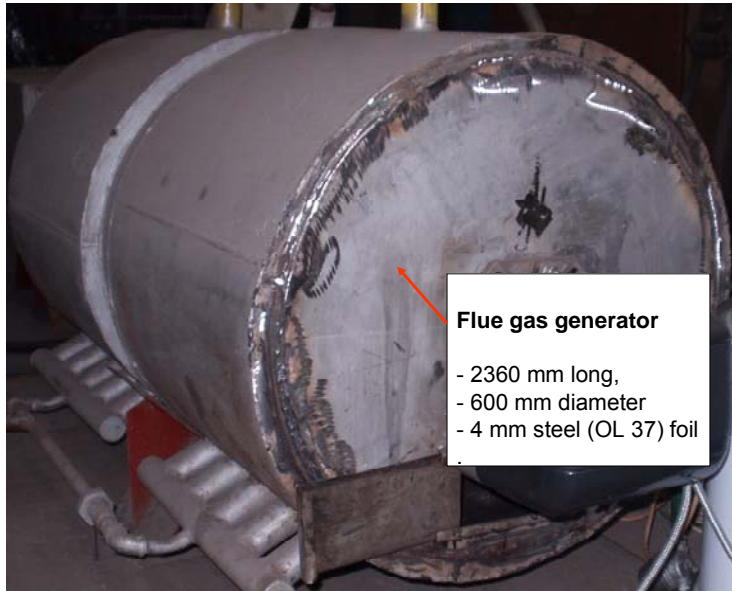
Combustion gas generator –frontal view
